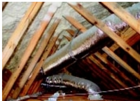
Both types of SPF can work well in most attics and cathedral ceilings without the need to ventilate (although one should follow the manufacturer's instructions). However, ventilation ducts can maintain desired temperatures more efficiently because they are in a conditioned space.
