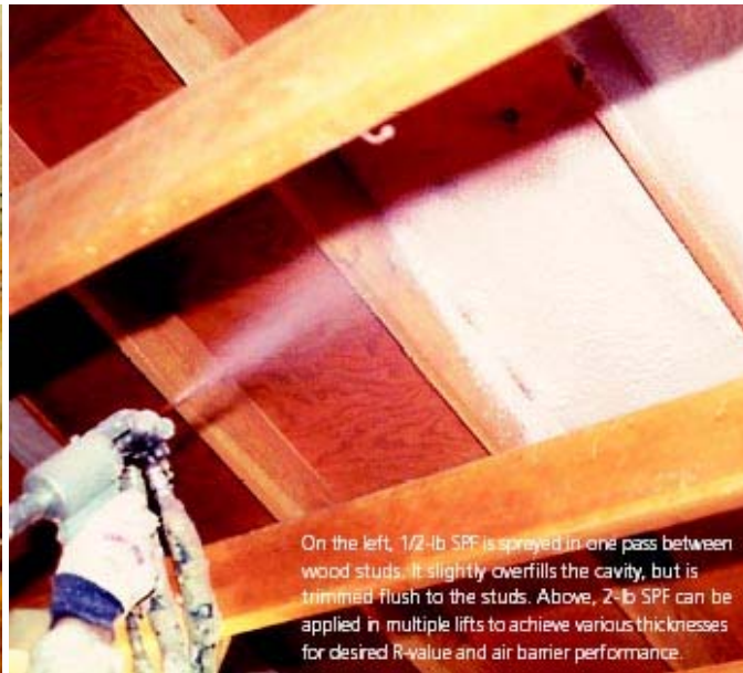
Left, 1/2-lb SPF is sprayed in one pass between wood studs. It slightly overfills the cavity, but is trimmed flush to the studs. Right, 2-lb SPF can be applied in multiple lifts to achieve various thicknesses for desired R-value and air barrier performance.
