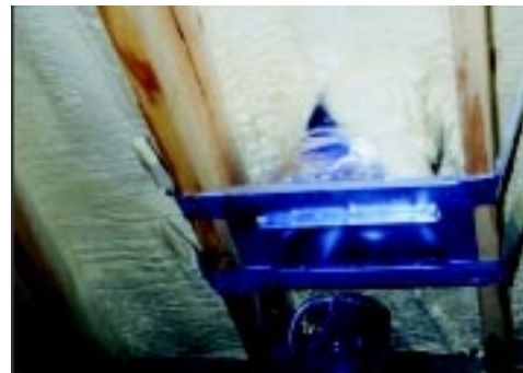
Both types of SPF can work well in most attics and cathedral ceilings without the need to ventilate (although one should follow the manufacturer's instructions). However, ventilation ducts can maintain desired temperatures more efficiently because they are in a conditioned space.
