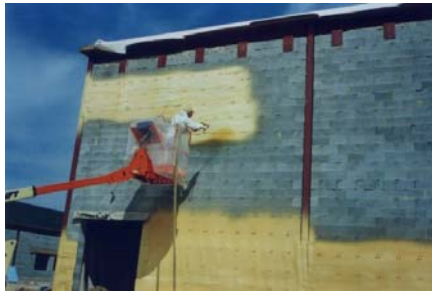
In the above curtain wall (CW) construction, 2-lb SPF is used to insulate the exterior of a building, helping to eliminate thermal bridging, while adding a secondary barrier against water penetration to the inside of the building. On the right, 2-lb SPF is used to achieve high R-value in a limited space.
