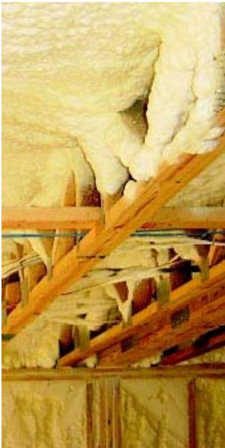
Left, 1/2-lb SPF is sprayed in one pass between wood studs. It slightly overfills the cavity, but is trimmed flush to the studs. Right, 2-lb SPF can be applied in multiple lifts to achieve various thicknesses for desired R-value and air barrier performance.
