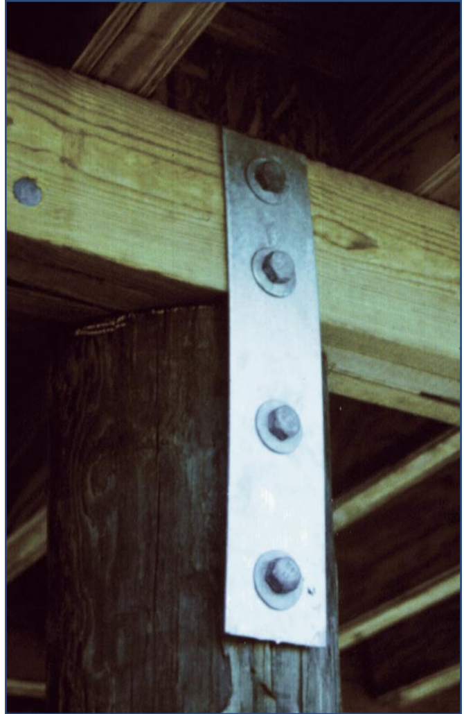
Metals corrode at a much faster rate near the ocean. Always use well-protected hardware, such as this connector with thick galvanizing. (For information about pile-to-beam connections, see Fact Sheet No. 13).
