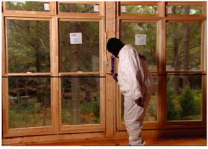
We completely seal the envelopes around windows and doors to prevent air leaks.
