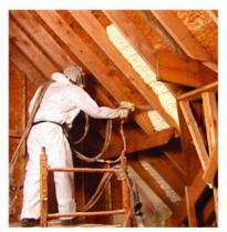
Airtight SprayFoam's versatility makes it a good choice to totally seal the envelope for a comfortable living environment. Here the underside of the roof sheathing is being sprayed.
