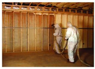
The solid nature and sealability of cured foam, which is moisture resistant itself, inhibit moisture-driven elements, providing for dry, comfortable interiors. There are many other advantages inherent to Airtight SprayFoam®: it helps reduce exterior noise, creates a barrier against gas and odor, retards insect and rodent penetration, and the strong, rigid, lightweight envelope of cured foam adds to the structural integrity of the house.
