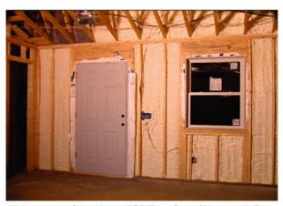
Using a combination of SPF and caulking, a tight seal can be made for a well-sealed envelope.
